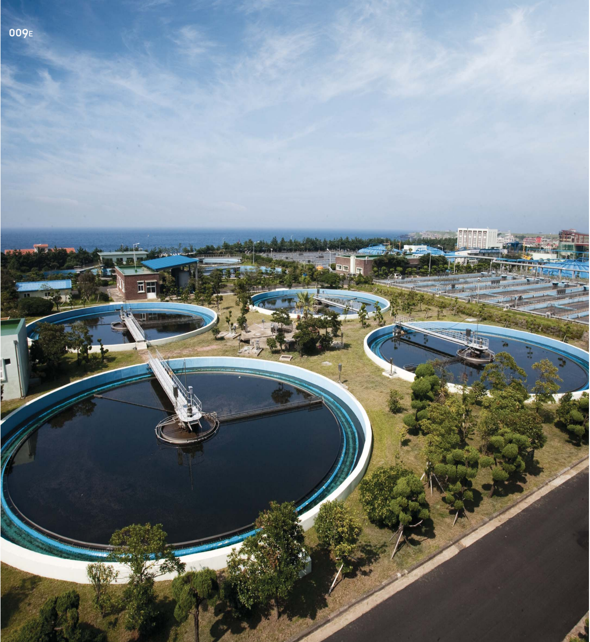
009E Jeju Advanced Sewage treatment plant Location: Jeju, Korea - Advanced Sewage Treatment: 130,000 m 3 /day - CNR Process Project period: 2006. 09 ~ 2009. 05
